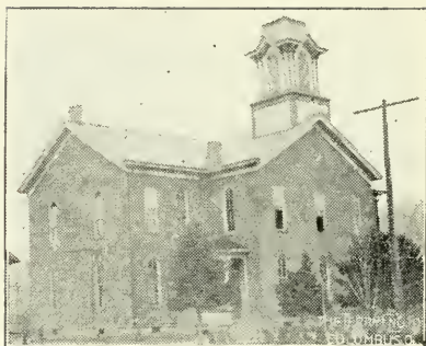
MAGNOLIA HIGH SCHOOL, OLD BUILDING.
